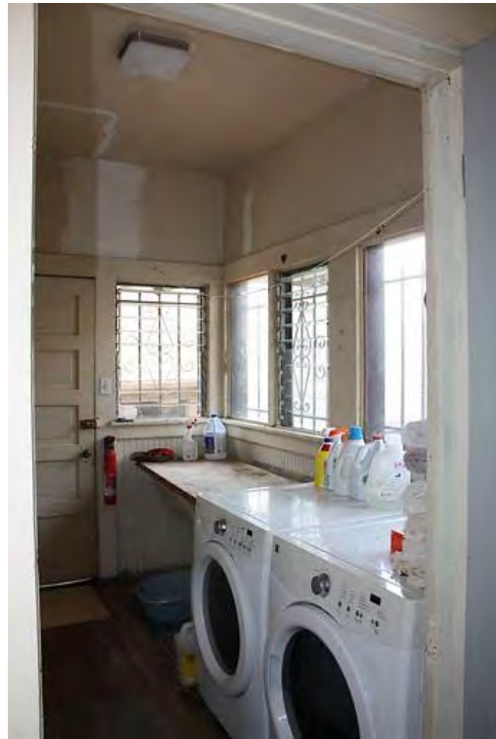
Laundry room, west off kitchen, former service porch: 5-panel door in west wall to exterior; wainscot of narrow tongue and groove; run of original window openings some with substituted glazing; original twin laundry sinks, covered at northwest corner, view west.
