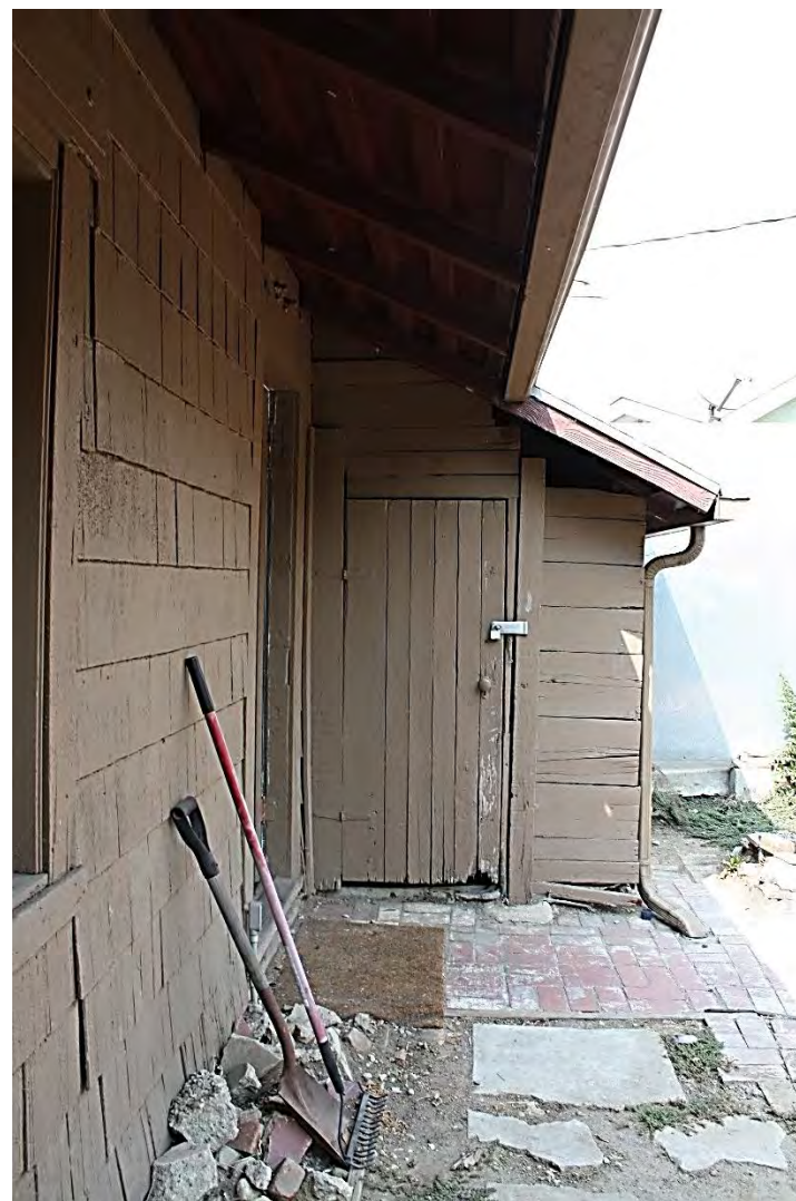
East elevation of "L" shaped garage: Main body beneath north/south gable at west, head of "L" at north, original shingle cladding, with small patch, and door, overhanging eaves with plain brackets, view north.
