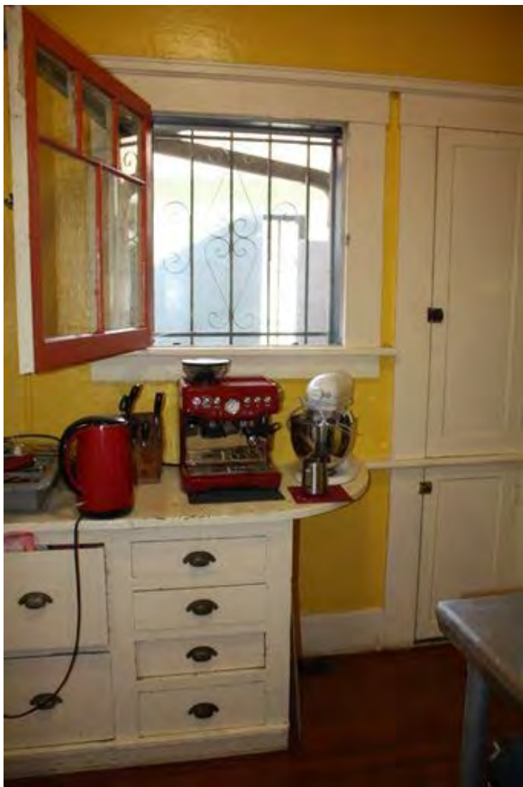
Pantry: Northwest corner, kitchen entry; original cabinetry, casement window, built-in cabinetry, north wall; corner of east work area, view north.
