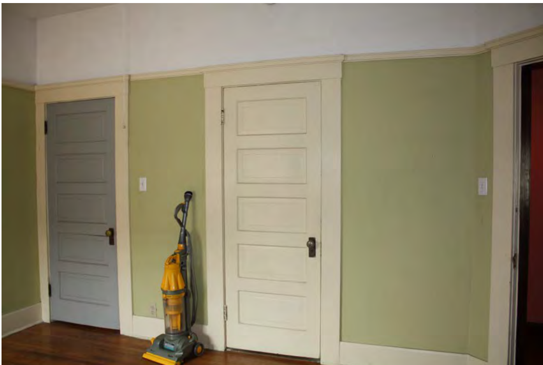
Original south home office, at west of living room/inglenook: Northwest corner; 5-panel door to private hallway at south of dining room breakfront, door in diagonal wall to short hallway north of living room with visitor's bench; original picture rail and baseboard around entire room, view north.
