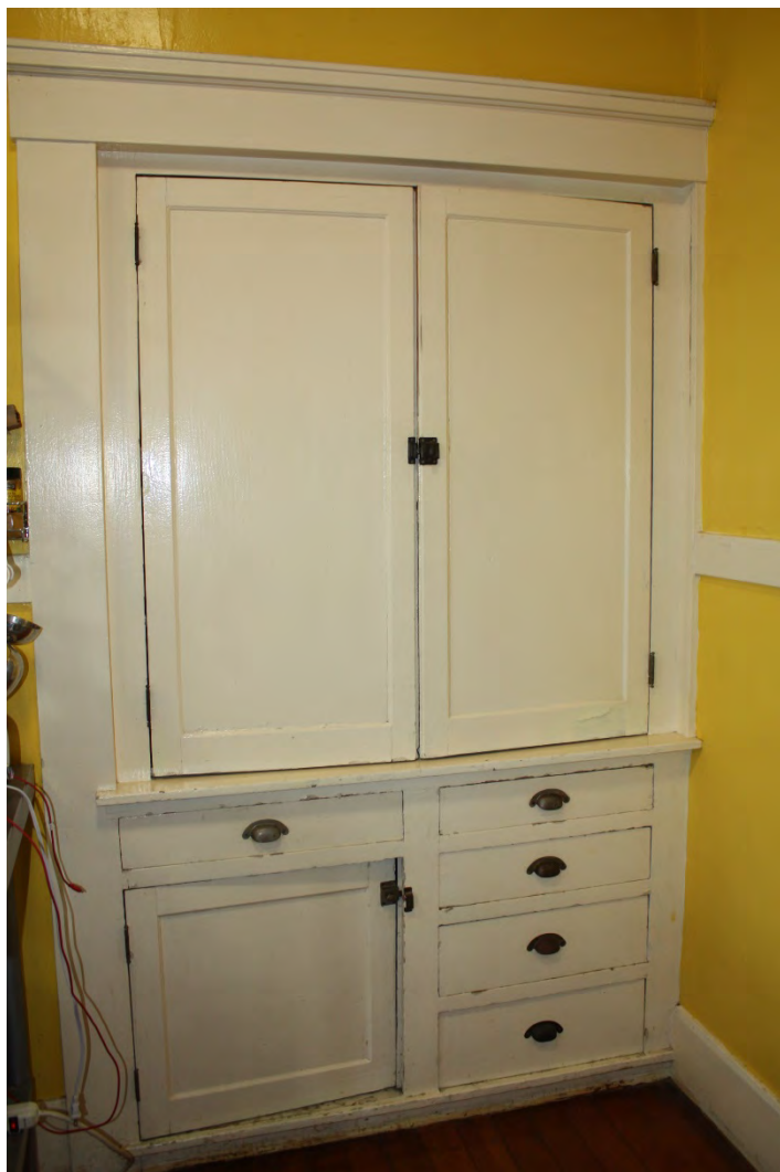
Detail: Original built-in kitchen cabinets and drawers, Southeast corner of kitchen, view east.
