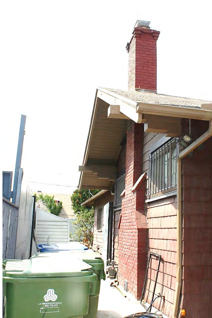
South elevation: Cantered wall in south protruding gable with inglenook chimney, overhanging eaves, tri-cut brackets, paired casement multi-pane windows, continuation of major east/west gable, south concrete driveway, southwest corner rear/west yard, view west.
