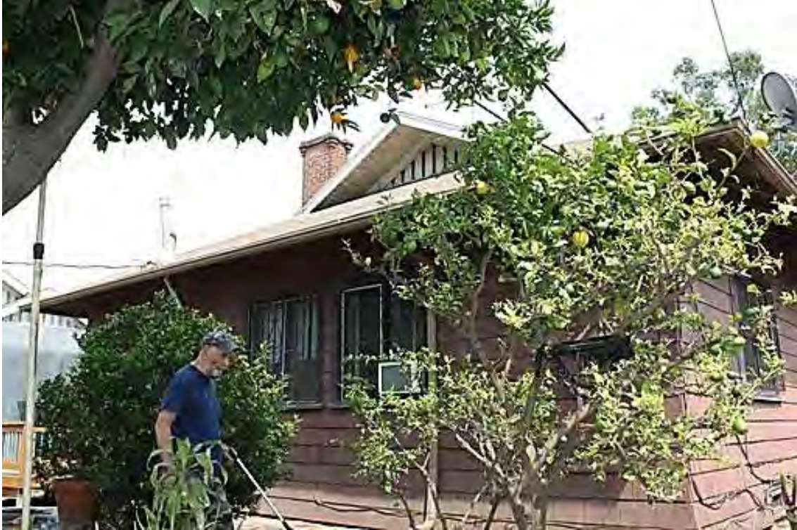
Rear/east elevation with kitchen chimney; southeast corner with canted walls; fruit trees, view northeast.
