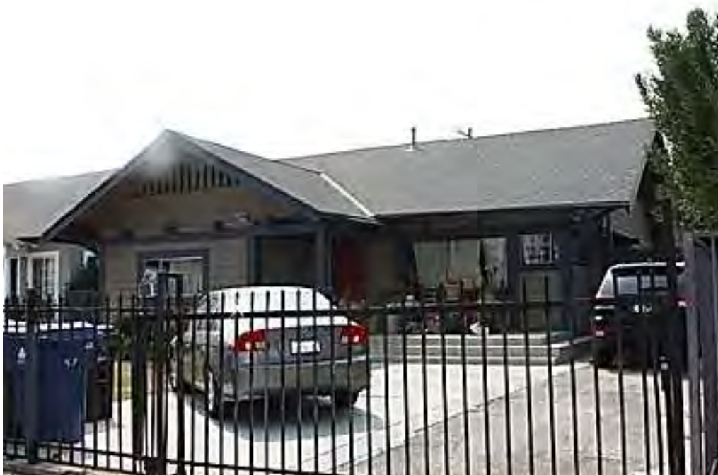
Craftsman Bungalow, altered, one of three-in-a-row on the west side of South Budlong Avenue, designed in 1908 by designers Barker & Weber for client A. C. Tobias, at 2921/south of 2915 S. Budlong Ave., the Subject bungalow.
