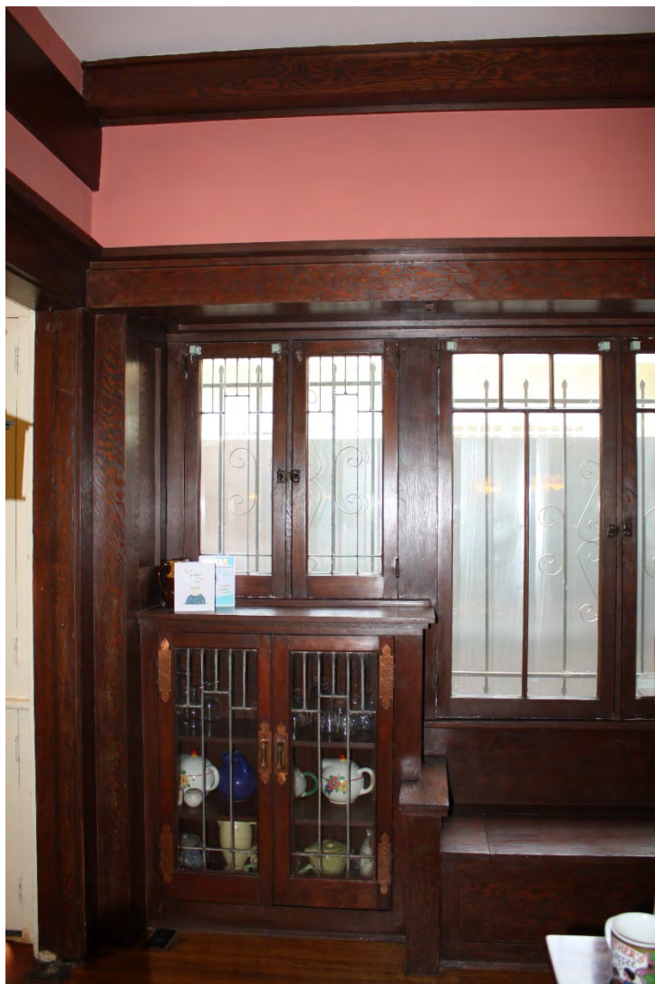
Dining room: West entry to pantry; built-in cabinets with leaded glass doors at each side of built-in bench, windows above cabinets patterned as cabinet doors, view north.
